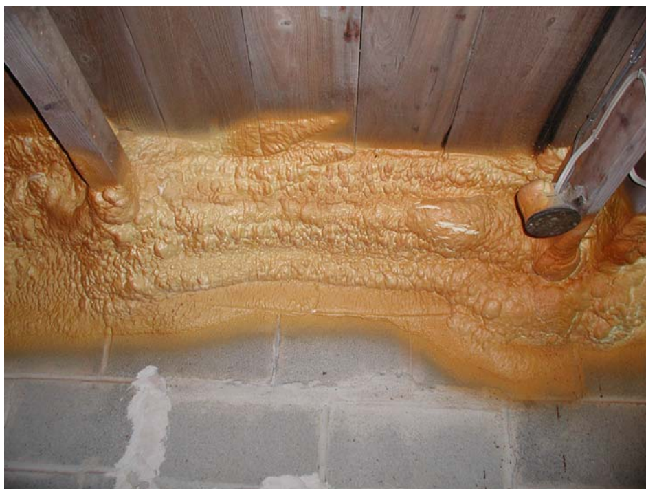
Figure 10. Rooms can be sealed with urethane insulation.
